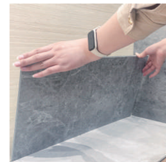
3. Install SPC wall panels
