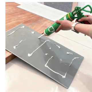
2. Gluing SPC wall panels
