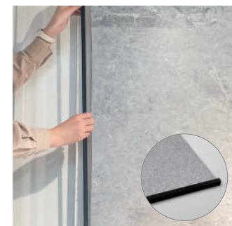
7. Installation completed the edge
